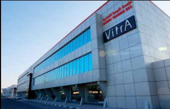
AIRPORT STREET BRANCH
